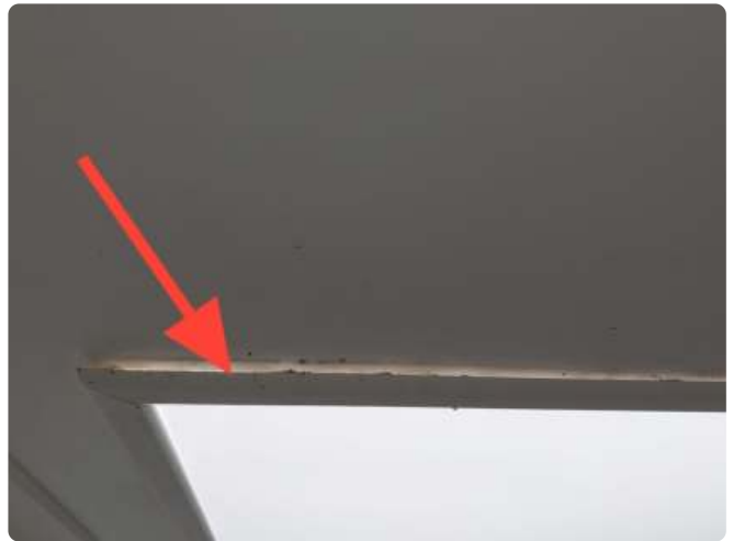
skylight frame separation
